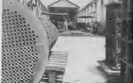
The Battlefield (7) stretches out at the west end of the shop building. Here tube bundles, foreground, are repaired and tested, and sent back to be put into use. This area will become a steel plate and structural steel storage area, and the bundle work will move into shop addition (9).
